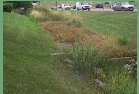
Example of an open channel retrofitted to provide better water quality treatment
