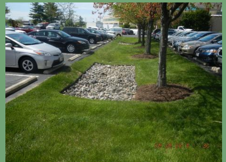
Example of a retrofit installed adjacent to large area of impervious cover
