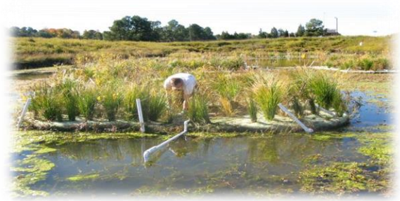
Regular inspection and maintenance is required to maintain FTW performance
