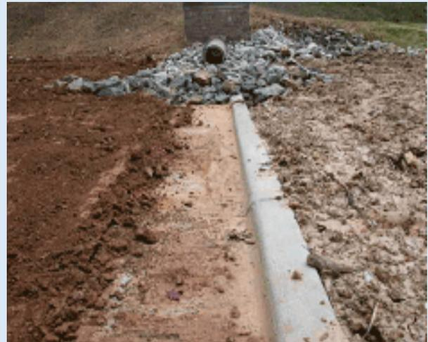
Figure 6. Level spreader just after construction
