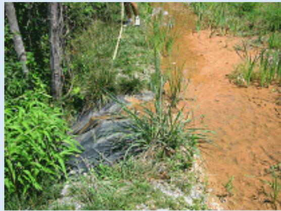
**Figure 3. Failure at level spreader constructed with ABC stone**
