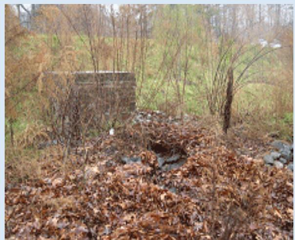
Figure 7: Sediment and debris build-up after approximately 4.5 years of operation
