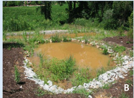
Figure 5. (A) Forebay schematic. (B) Image of level spreader with forebay
