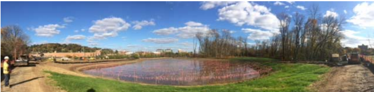
Four Mile Run Wetlands Restoration project completed in the Summer of 2016. The plants and grasses have since become established and grown in.
