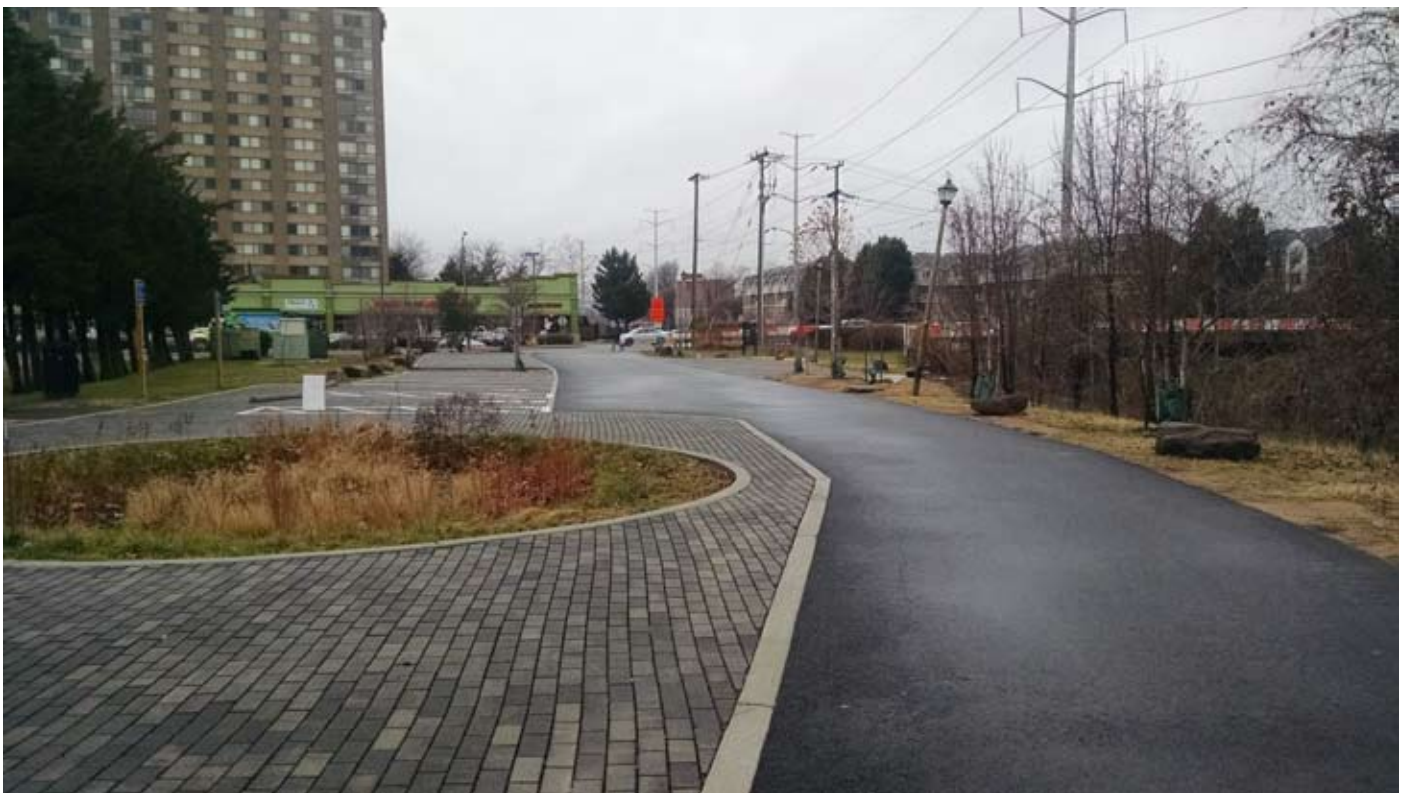
Four Mile Run newly restored partially permeable parking lot and rain garden.
