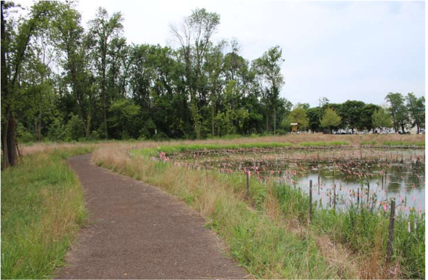
Porous pavement trail and restored wetlands.
