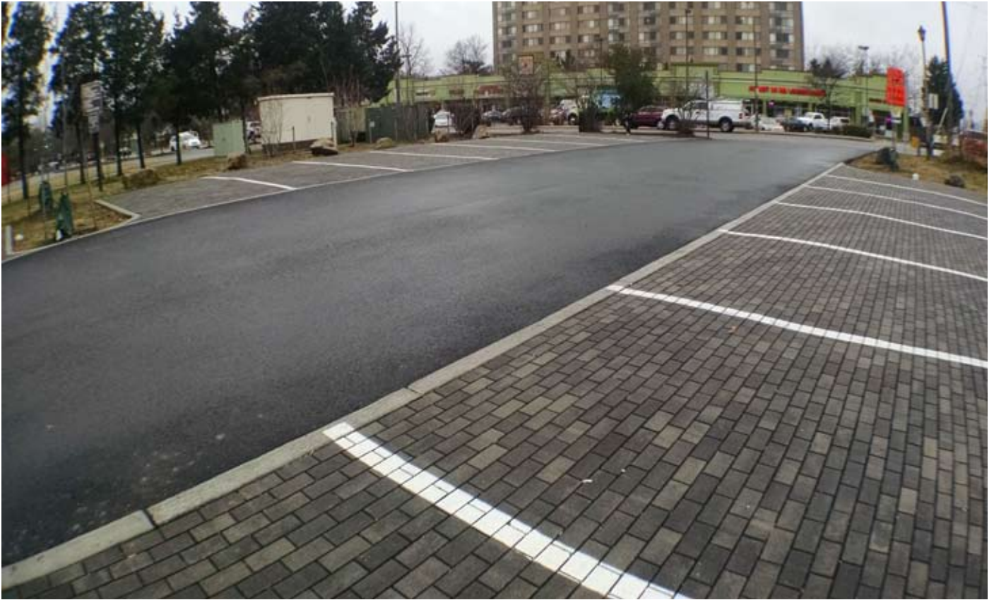
Newly renovated Four Mile Run parking lot with permeable parking spaces.
