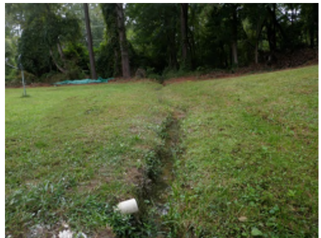
899 Tyler Drive: Upstream Location of RSC Channel Facing Northwest
