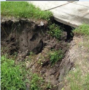
Inlet Erosion
