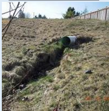
Inlet Erosion
