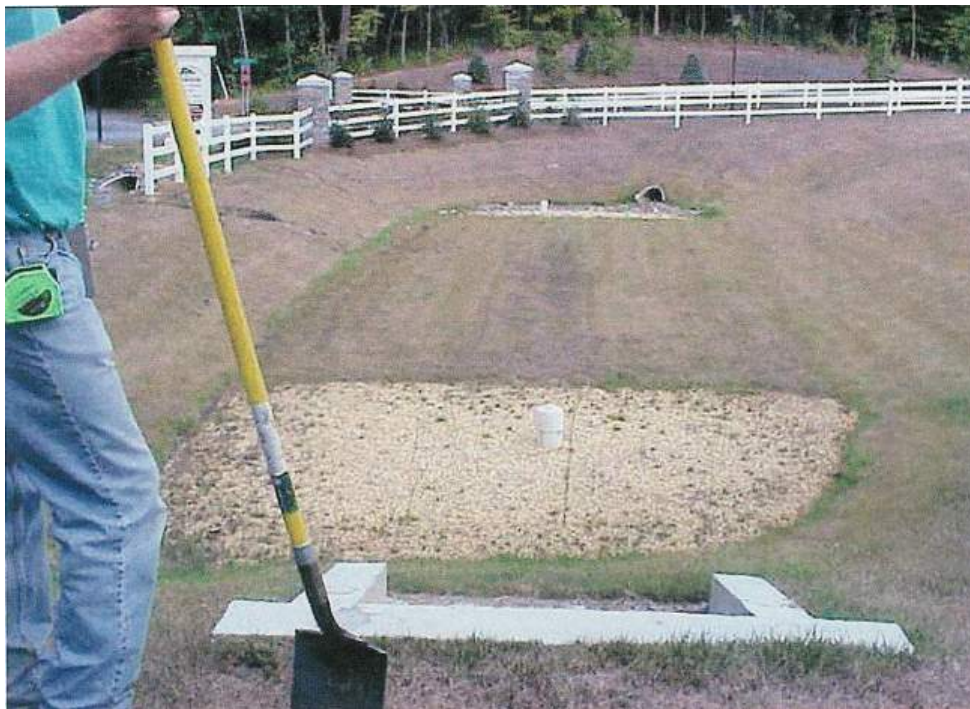
Figure 12.3. Hybrid Sand filter in a Detention Basin
