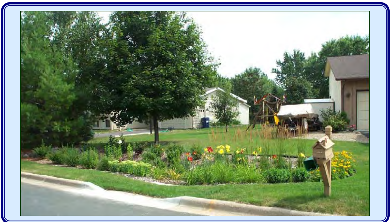
Photo 1: Typical Bio-infiltration 'Rain Garden'.
