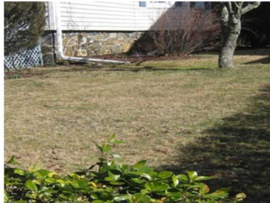
Runoff from both of these downspouts travels at least 40 feet over grass which will usually disconnects them unless your lawn is very steep, These disconnected downspouts are often a poor candidate for a rain garden
